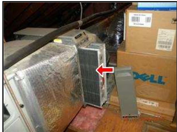
10.7 Picture 2 Electrostatic and Washable Filters
